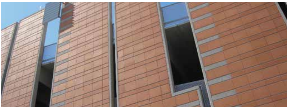
Figure 6b Close-up of terra cotta tiles. Photos: Fennick McCredie Architecture.
