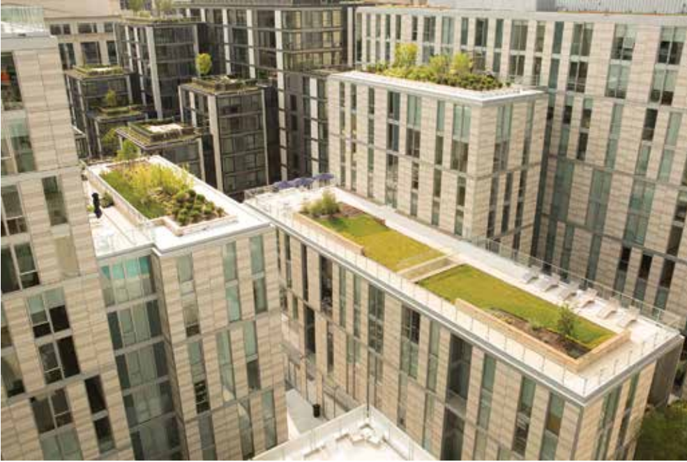
Figure 8a Overview of CityCenterDC, Washington, D.C.
