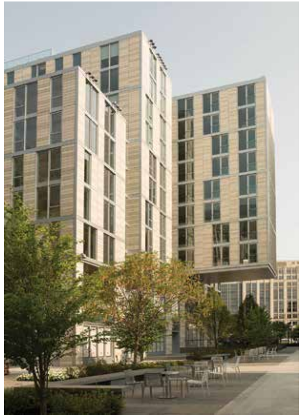
Figure 8c Precast panels shift from elevation to elevation.
