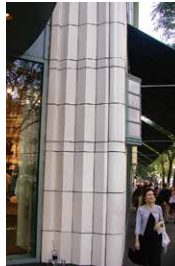
Figure 5b Flat, fluted, and round terra cotta tiles.
