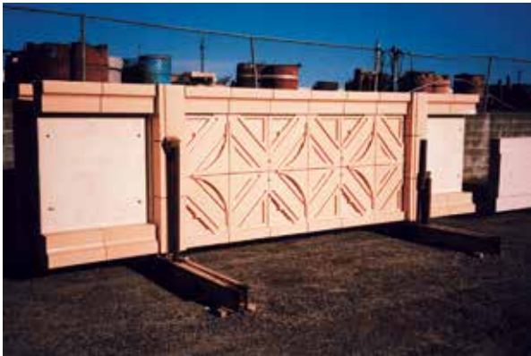
Figure 4b Terra cotta spandrel units.
