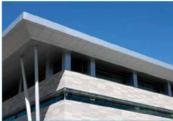
Figure 7c The high-performance precast concrete panels provided both energy efficiency and protection from ballistic penetration.
