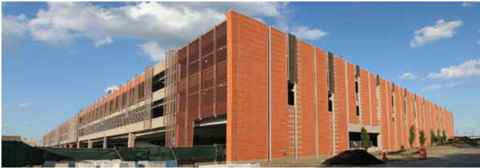
Figure 6a CONRAC at Logan International Airport in Boston, Mass.
