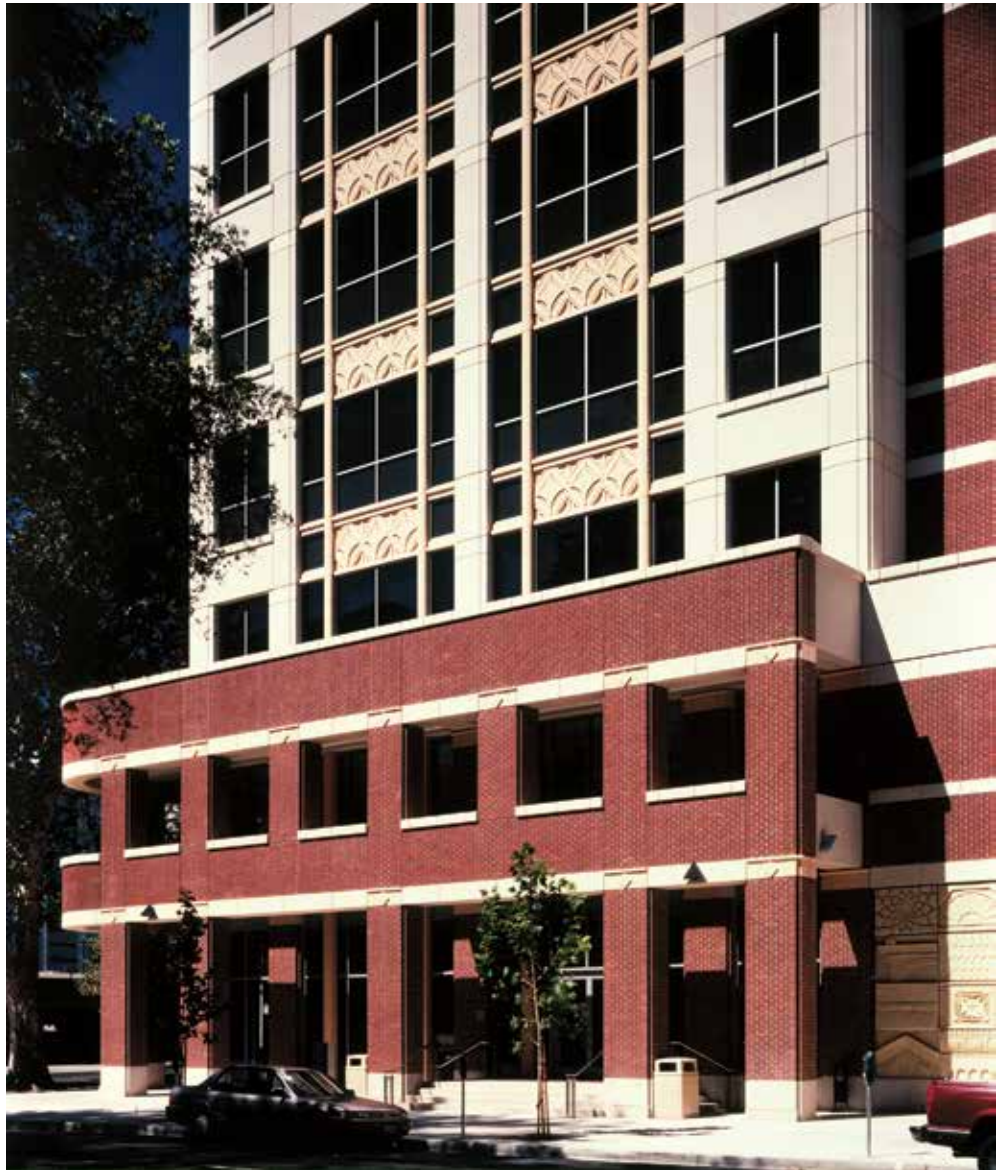
Figure 4a Sacramento County Systems and Data Processing Building, Sacramento, Calif. Photos: HDR Architecture Inc.
