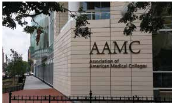
Figure 11c Nearly 5,800 pieces of 1 inch (25 mm) solid tiles were used in 13 different profiles and an ultra white color.
