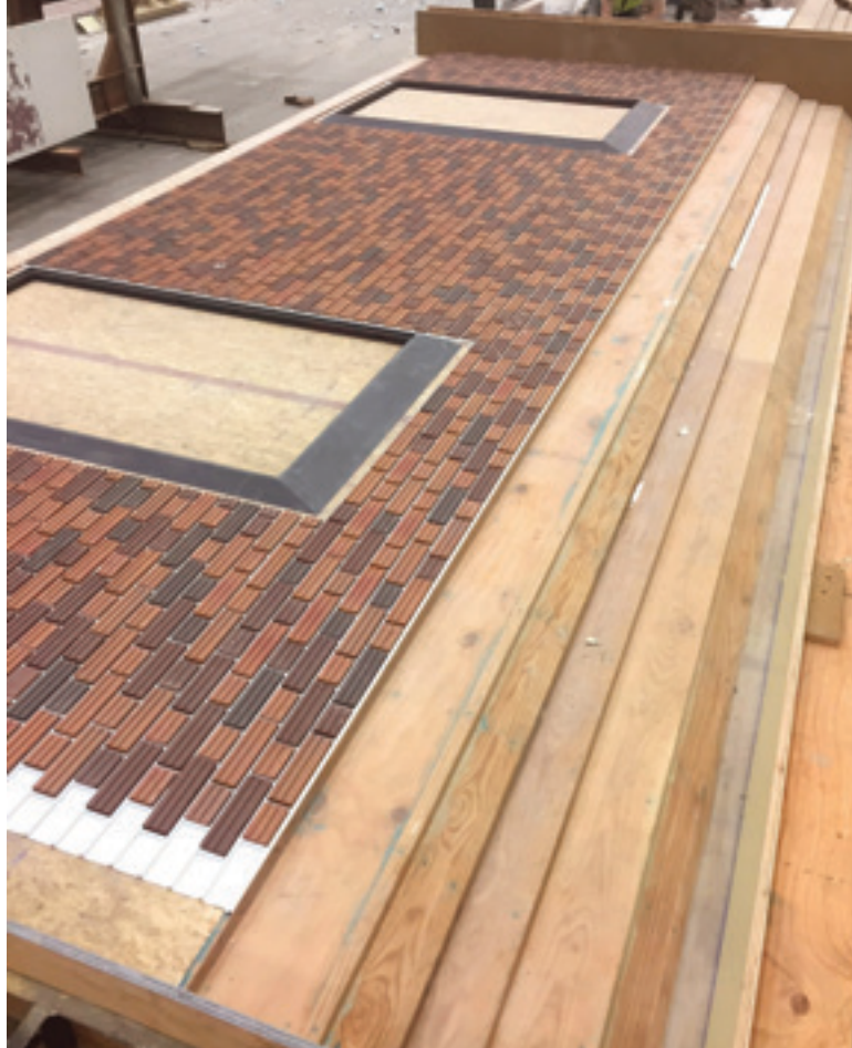
The casting of the wall panels for the Pioneer Hall project featured inset brick surrounding the 3-D printed blockouts that created the window shapes. Photo: Wells Concrete.
