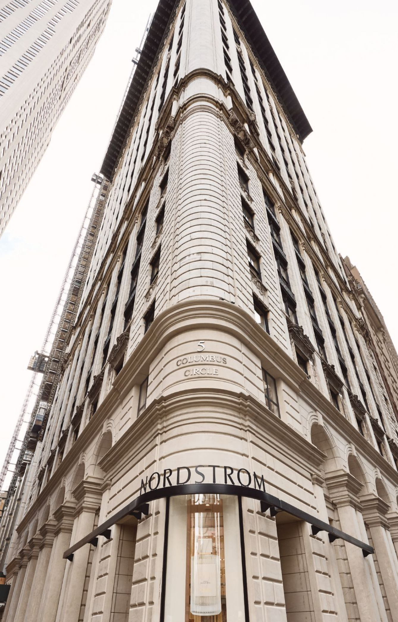
Gate Precast Company's plant in Ashland City, Tenn., was honored with the 2019 Sidney Freedman Craftsmanship Award for its work on the Nordstrom store façade in New York City. Photo: Erin Derby Photography.
