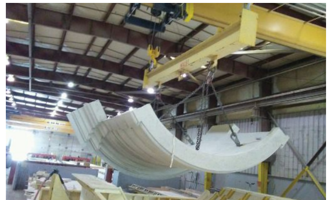
A crane lifts a piece of precast concrete at Gate Precast's plant in Ashland City, Tenn. Photo: Gate Precast Company.
