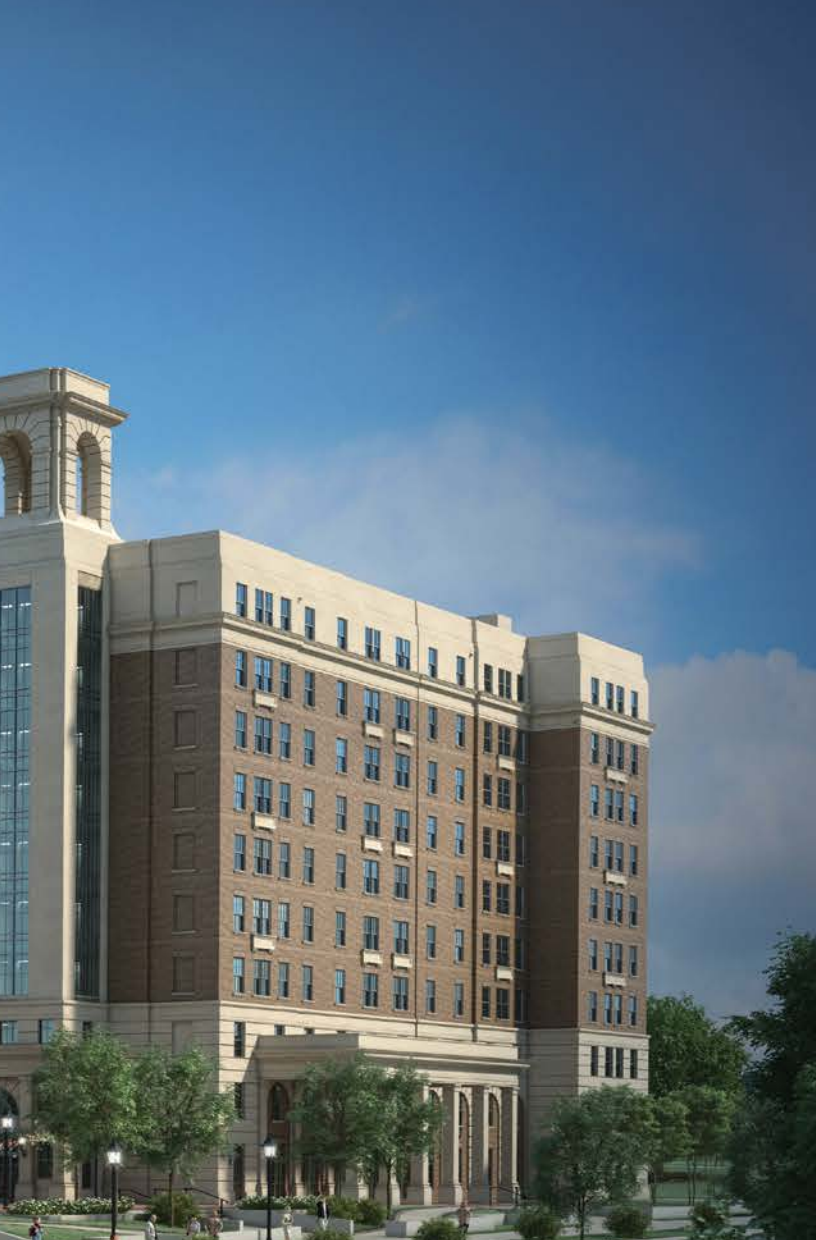
Several finishes, including inset thin brick, have been used on the insulated architectural precast concrete wall panels used on the new residential buildings at Longwood University. A variety of architectural ornamental pieces also are being cast. Photo: Gate Precast.
