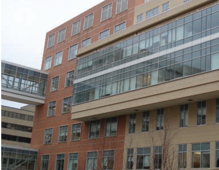
The University of Michigan Cardiovascular Center, Ann Arbor, Mich. PHOTO COURTESY OF THERMOMASS BUILDING INSULATION SYSTEMS
