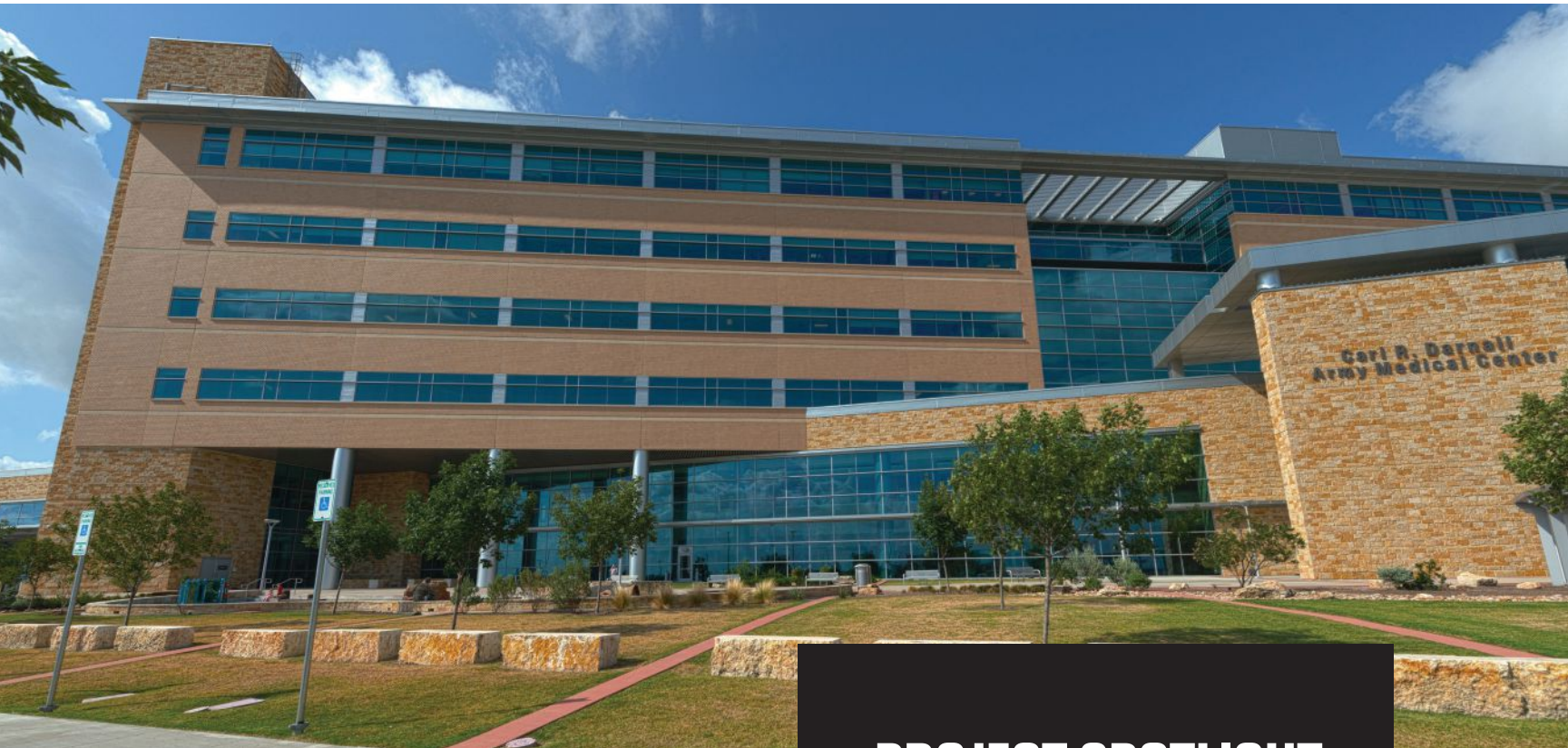
The Carl R. Darnall Army Medical Center at Fort Hood looks stunning with its façade of precast concrete and two-tone embedded thin brick. Photo: Nick J. Cool/The Image Works.
