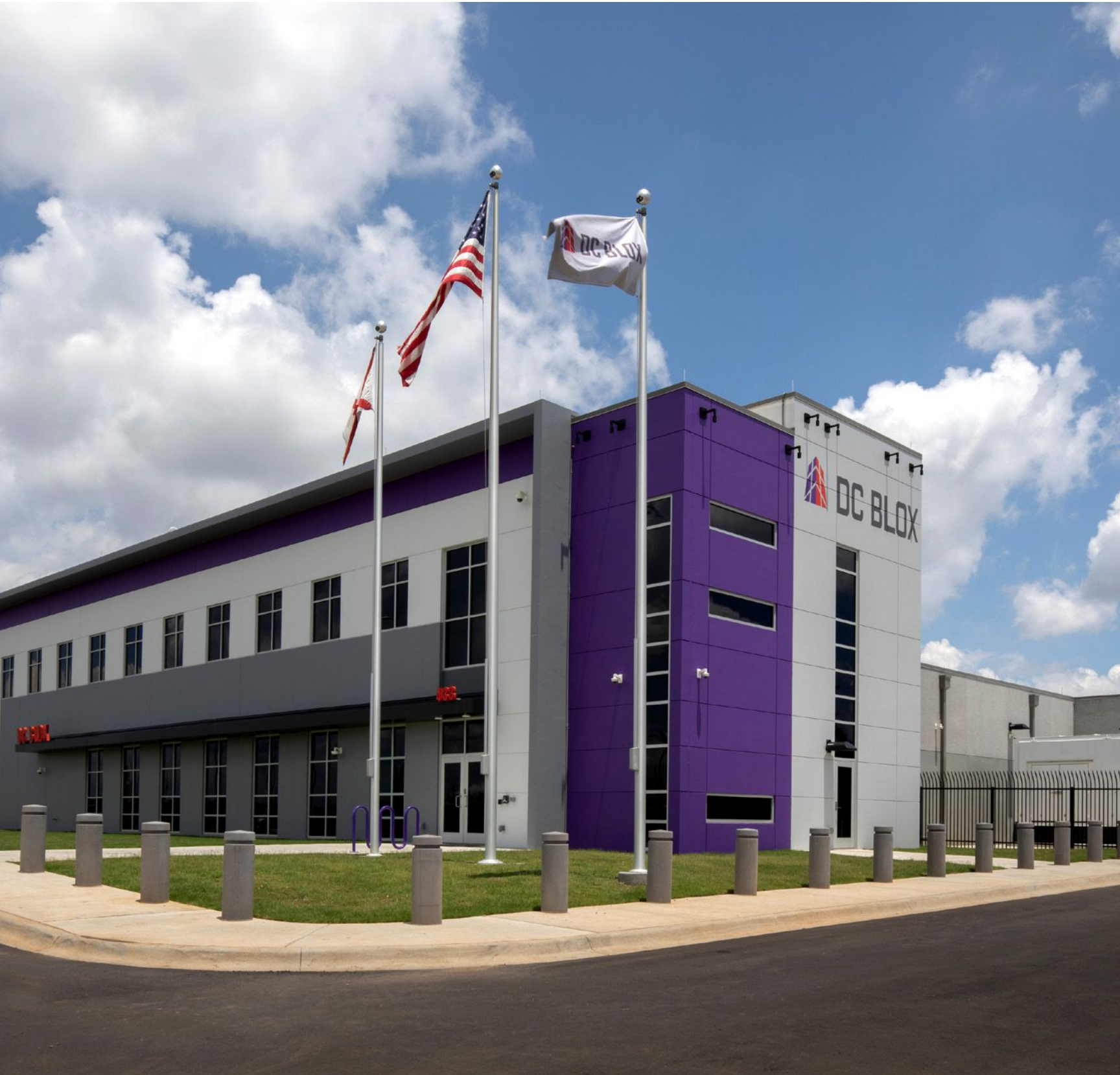
DC Blox in Birmingham, Ala., won a 2021 PCI Design Award for best data center. GATE Precast supplied the precast concrete. Photo: DC Blox.
